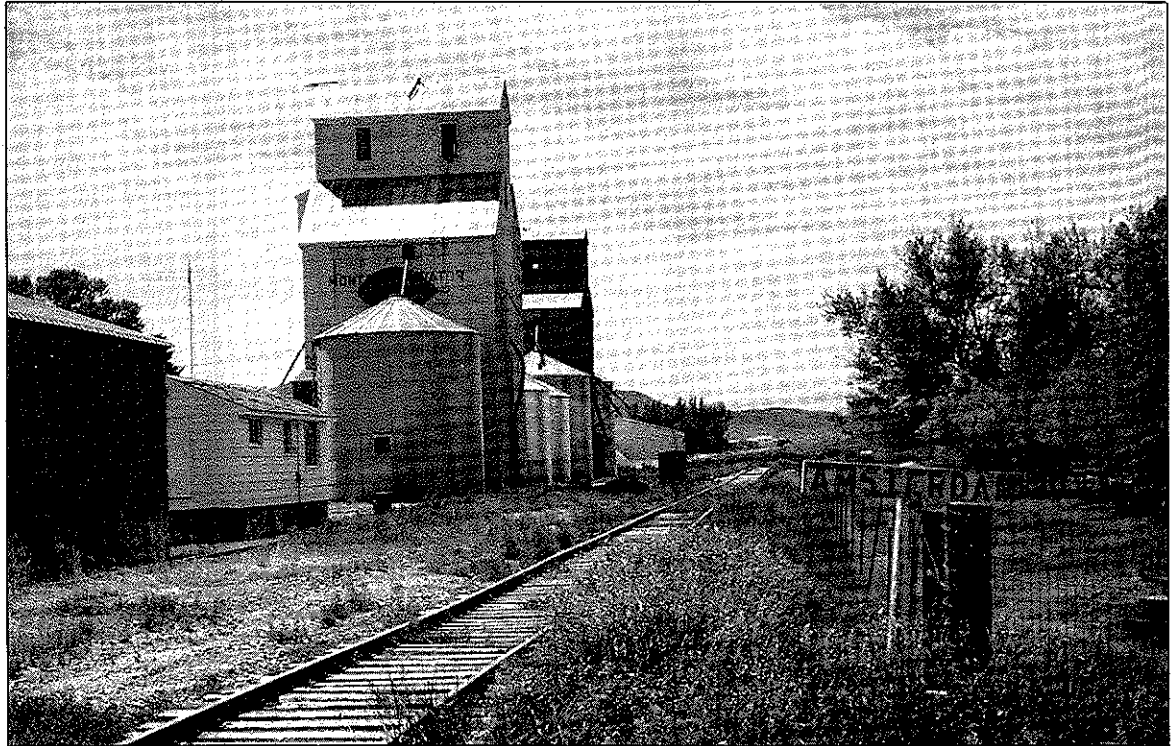
Grain elevator at "Amsterdam"
