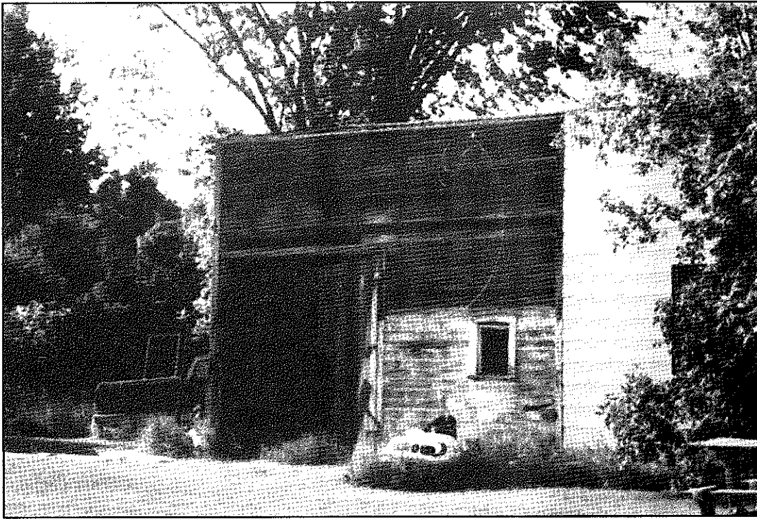
Commercial building, unoccupied, 1997.
