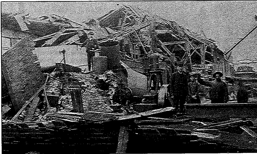
Ducey Lumber Company Mill in ruins, North Muskegon.
