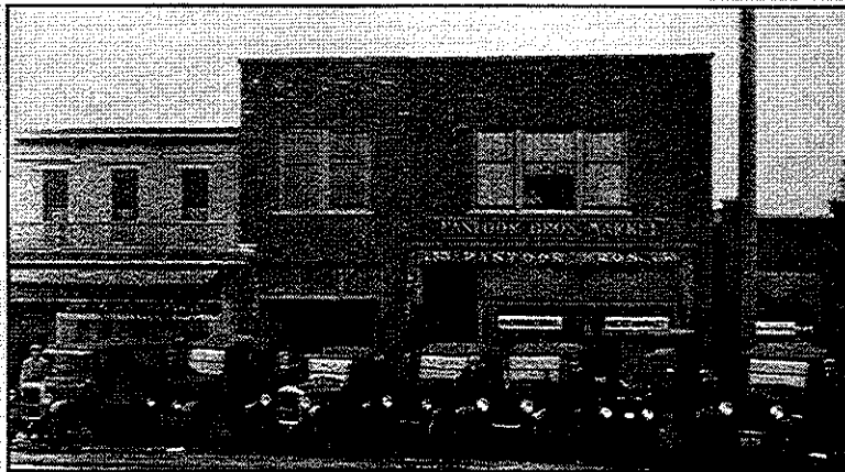
"New" Pastoor Brothers Market and the John G. Oom Hardware Store, circa 1925. The street numbering was changed and space between the buildings was enclosed. The front of the building was veneered with bricks, while additions were also made to the rear of the building.
