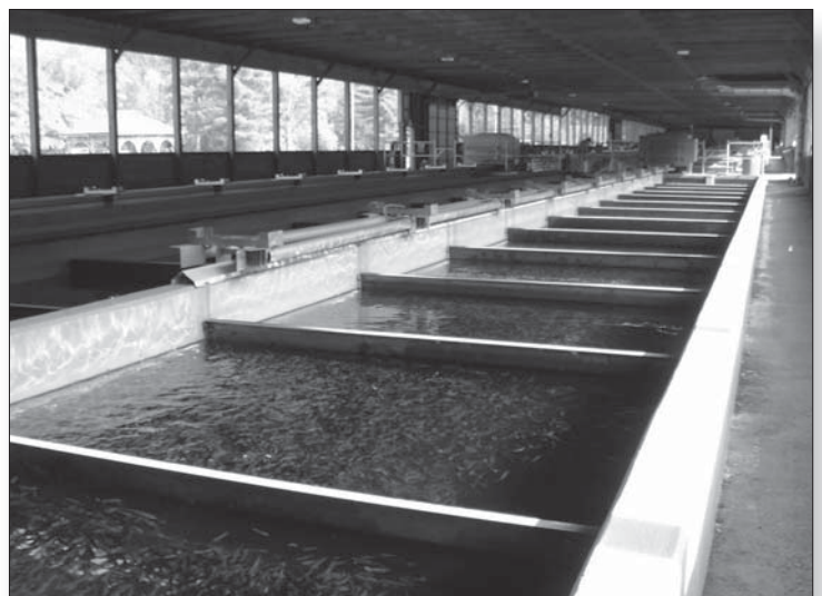
A concrete raceway at the Harrietta Hatchery, showing a series of baffles. Image courtesy of the Westers family.
