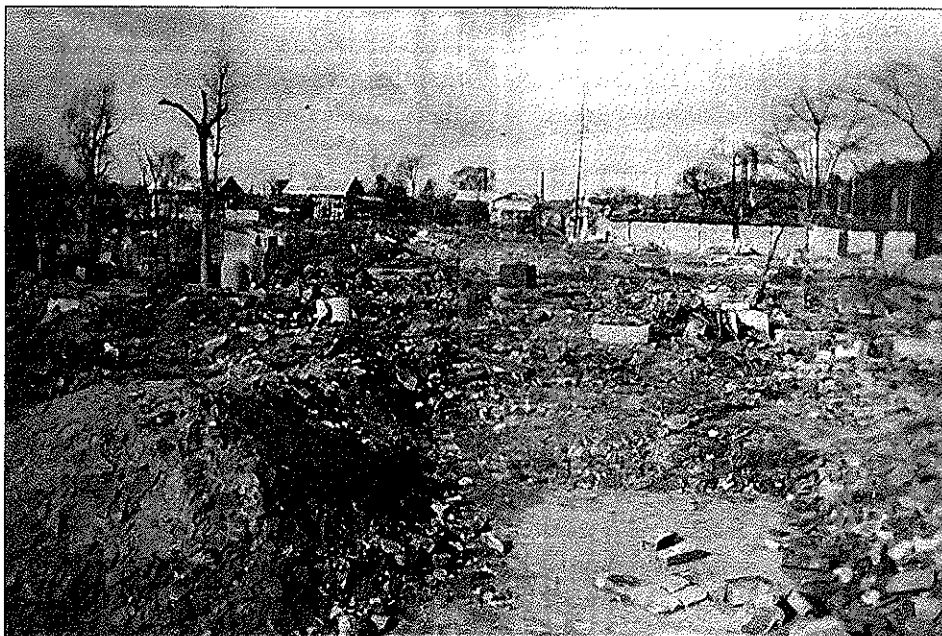
Damage at Matsuyama near Kochi. Photo: Courtesy of the author.
