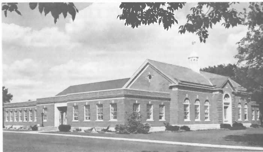
Views of Hekman Memorial Library with Reading Rooms
