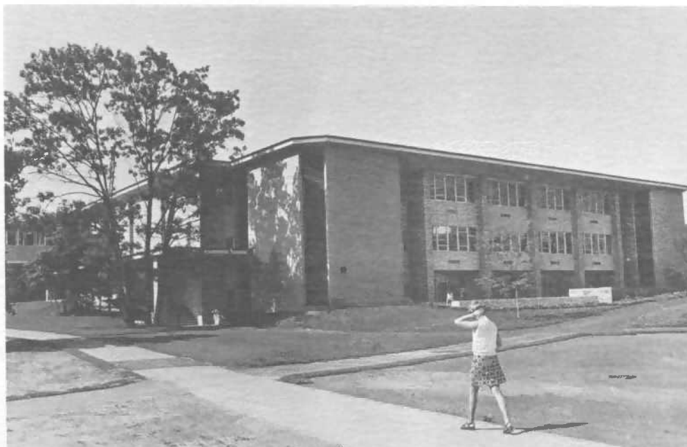
New Library addition. Lower level is below the three floors on the picture. The building is constructed to support an additional floor if necessary in the future.
