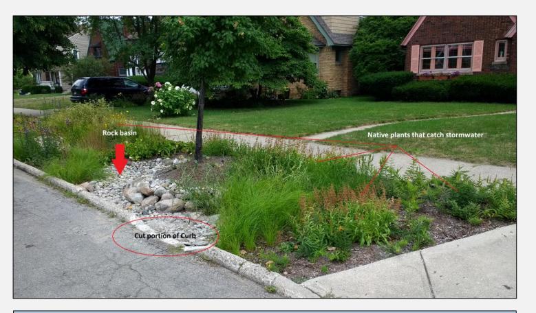
Figure 1: In a curb-cut rain garden stormwater runoff enters into a rocky basin through a literal cut in the curb; native plants assist in filtering and evapotranspiring the trapped rainwater.
