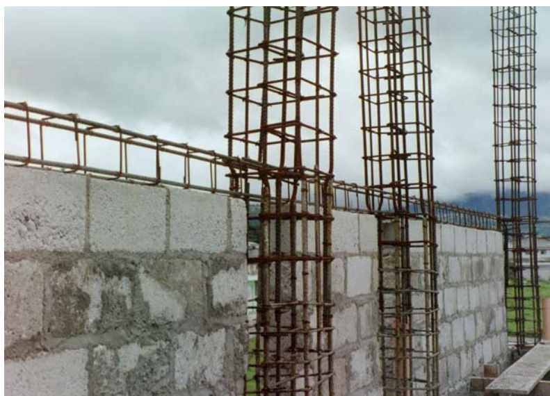
Figure 5: Close-up of Rebar Cages of Vertical and Horizontal Reinforcing
