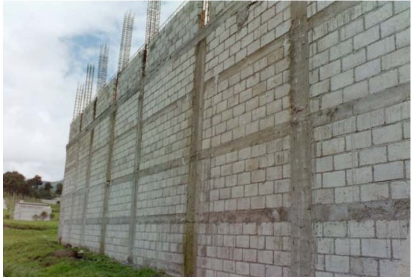
Figure 4: Vertical and Horizontal Reinforcing
