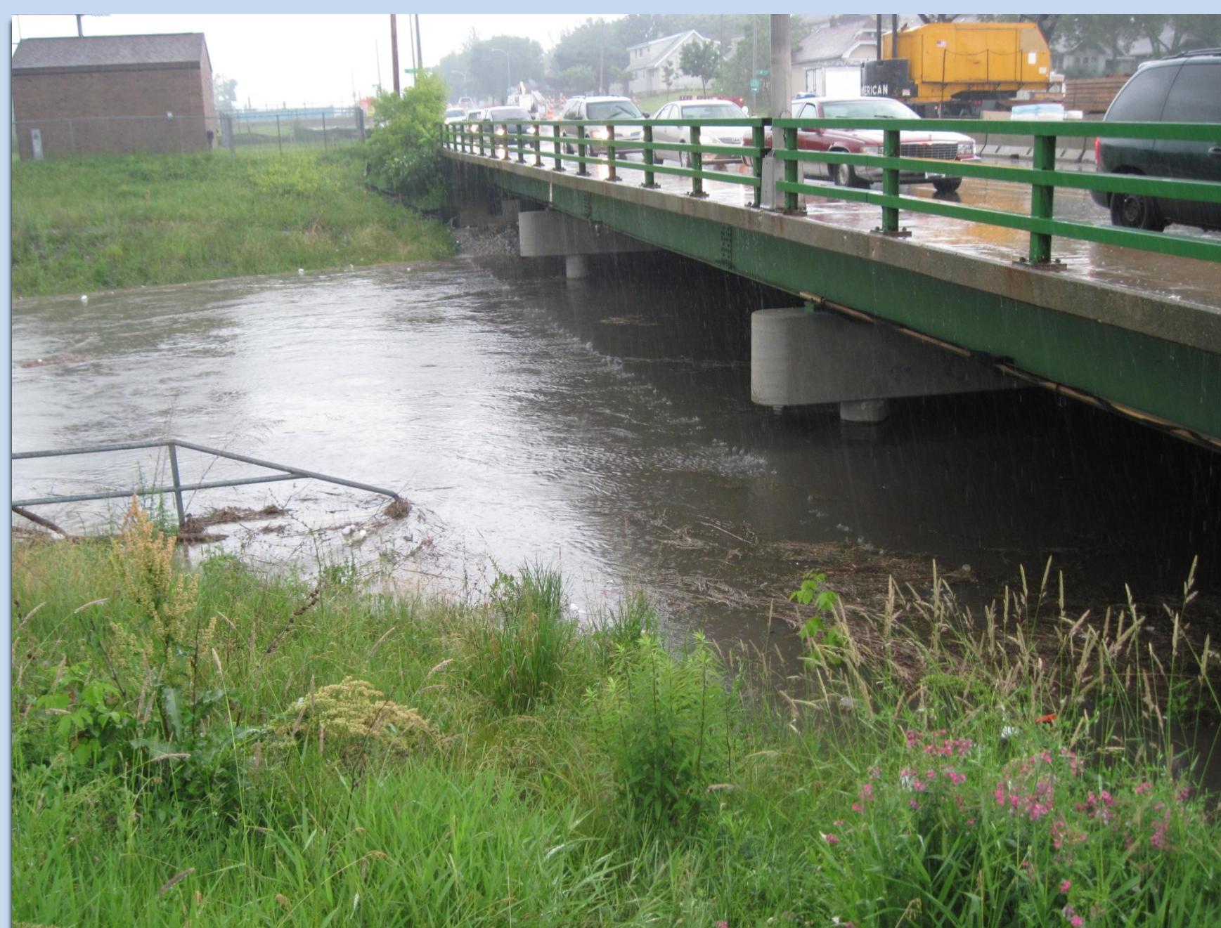
Figure . A bridge after one of the heavy rainfalls.
