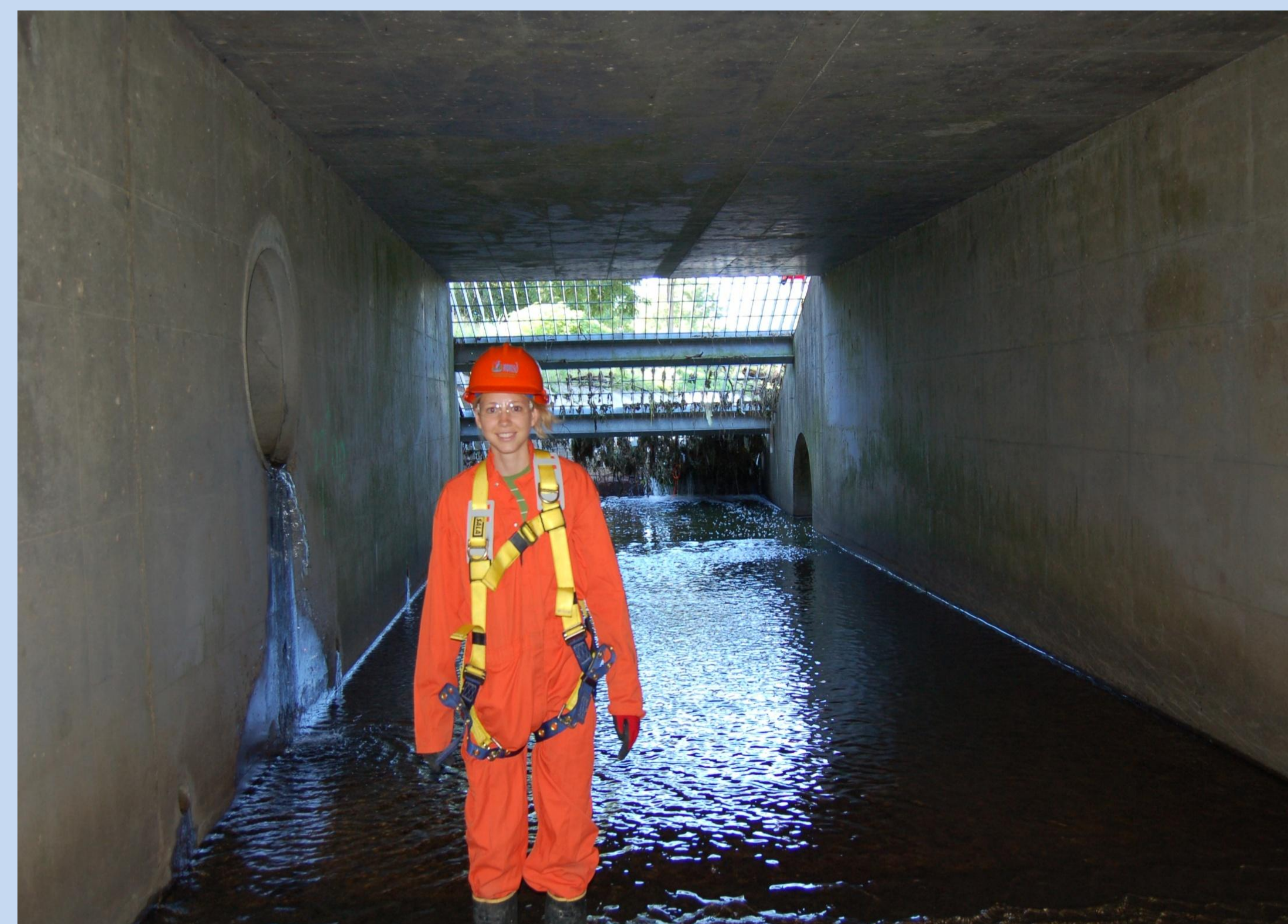
Figure 3. Inside a box culvert for an inspection..
