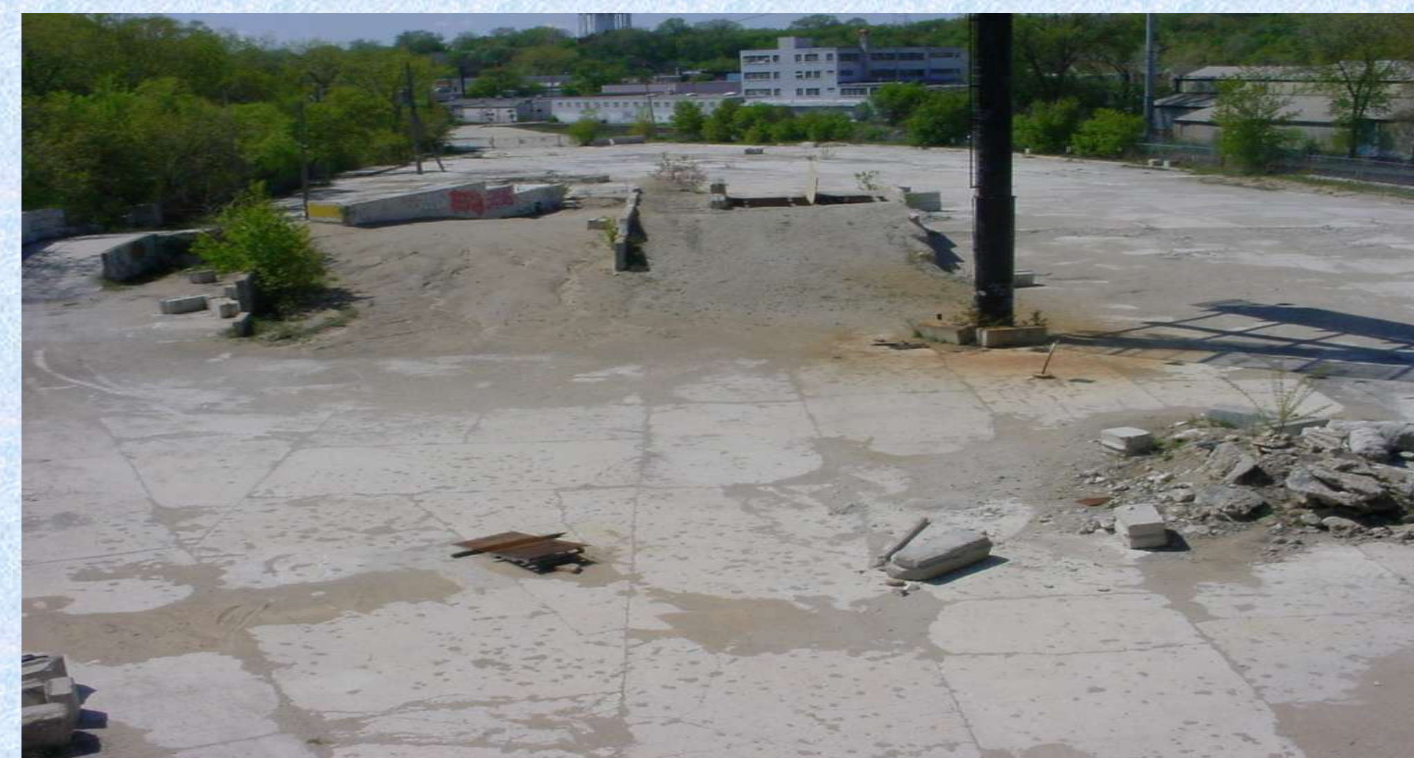
Figure 2. The soil contamination project before work began at the site.
