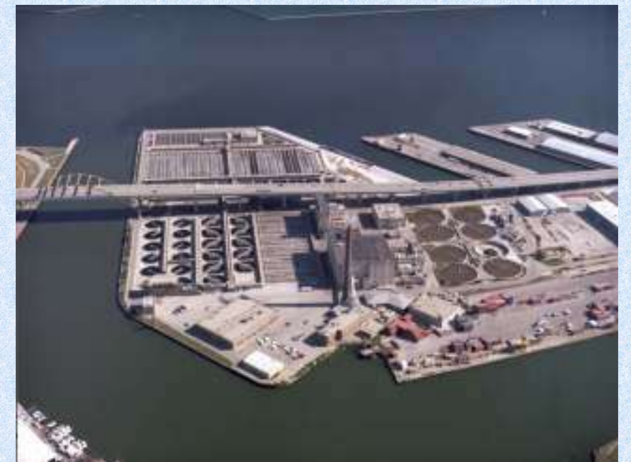
Figure 4. Jones Island Sewage Treatment Facility.
